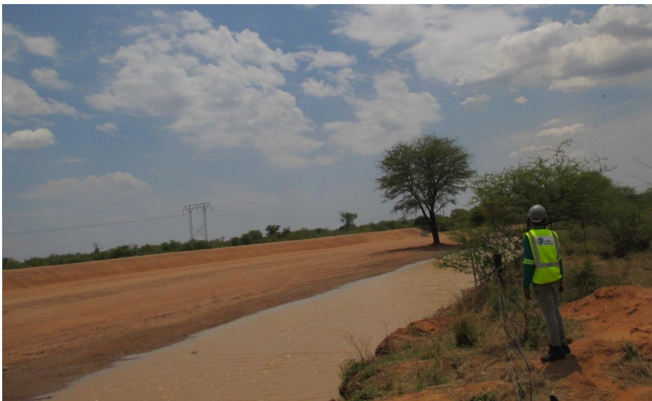
Figure 13: Unlined clean water diversion channel at Medupi
